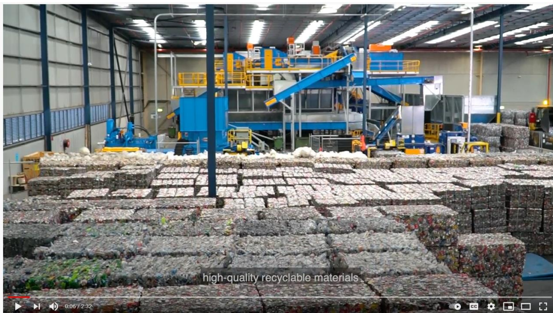
Cleanaway's Container Sorting Facility
