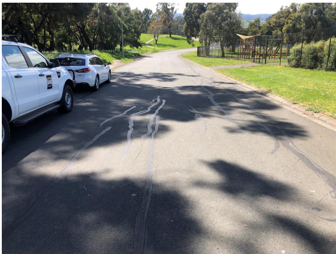
Figure 3-12 Sealed cracking within existing road east of site
