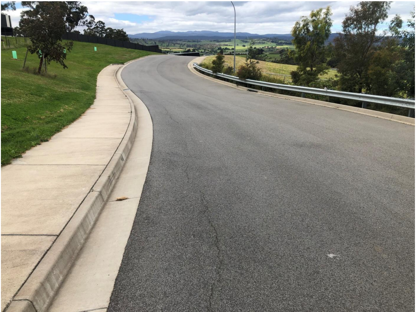
Figure 3-13 Longitudinal cracking within new road south of site
