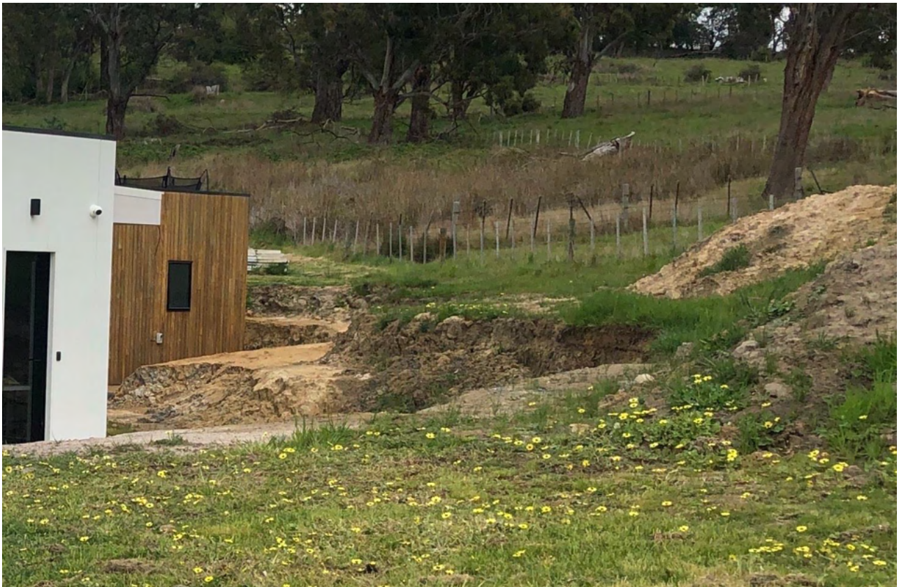
Figure 3-15 Cut batter failures on slope south of site
